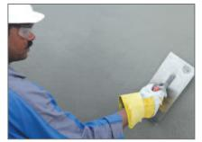
applied on the prepared block work and fair faced concrete surface. A rough texture has to be obtained to provide a mechanical key for the subsequent coat of CP2 LGT.
